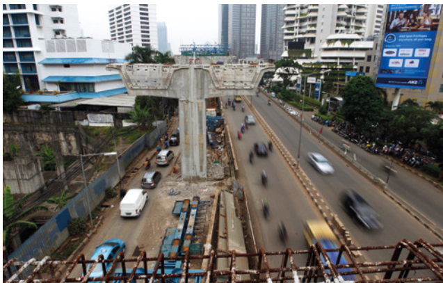
Vehicles drive past the construction site for a new highway in the business district in Jakarta. Despite claiming it will be completed by June this year, it will not be open for months.
